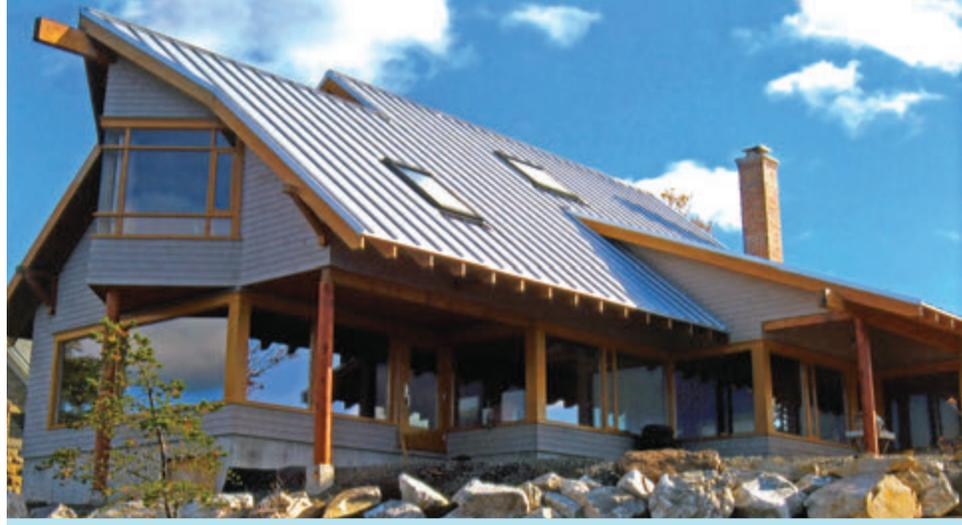
*The Heritage™ Series steel panels are offered in standard widths of 20 1/4" or 16" — to suit and adapt to any style of sloped roof and to enhance any building architecture.*
